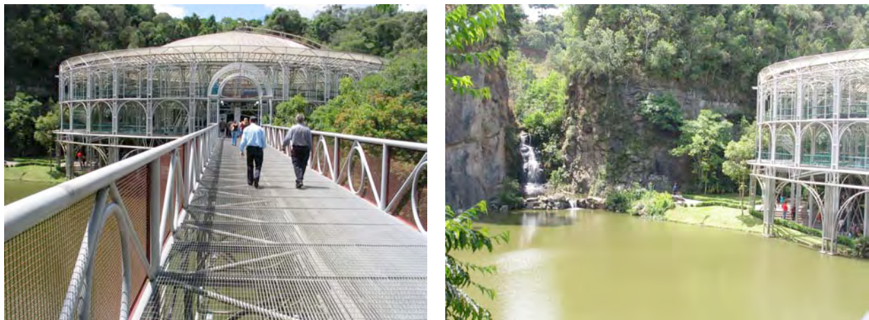
Figure 15. Opera House built in two months out of recycled metal piping in an old quarry
